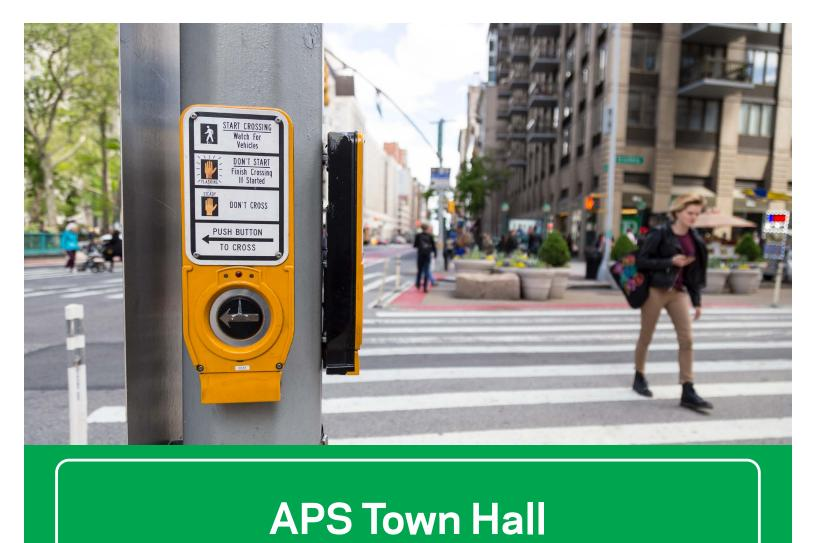
Accessible Pedestrian Signals (APS) are devices affixed to pedestrian signal poles to assist blind or low vision pedestrians in crossing the street. APSs are wired to a pedestrian signal and send audible and vibrotactile indications when pedestrians push a button installed at the crosswalk.
